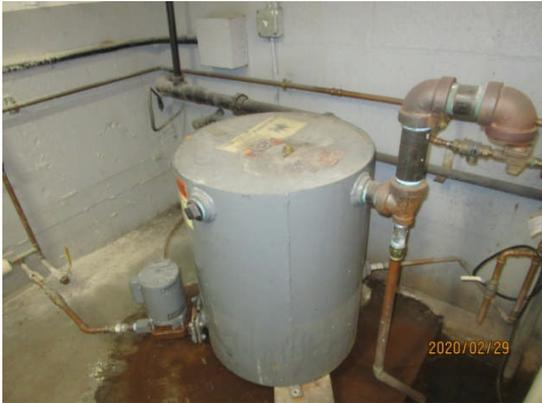
Condensate pump needs repair, leaking
