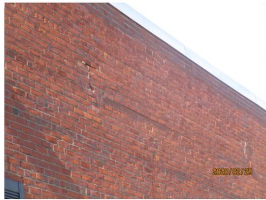
bulging and cracked bricks
