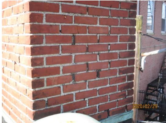
loose mortar joints chimney
