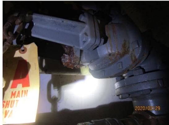
leaking main sprinkler valve, corrosion
