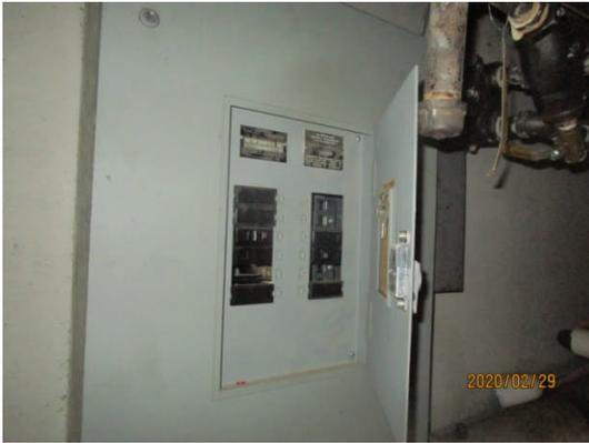
Old electrical panel, missing knockouts
