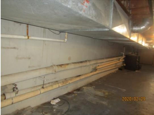
Cast-iron drainpipes, corrosion, pitting
