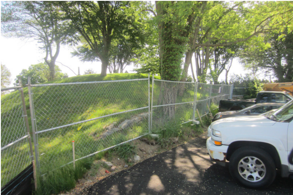
6. View of existing conditions at northwest corner of site.
