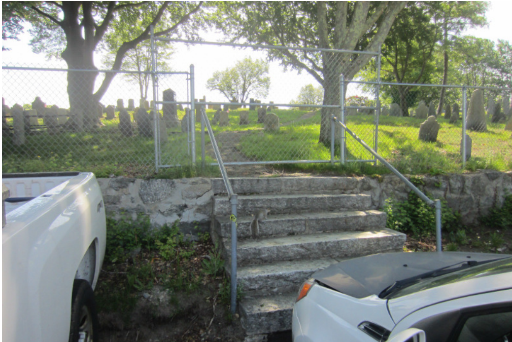
9. Existing stone wall and steps at east side of parking lot
