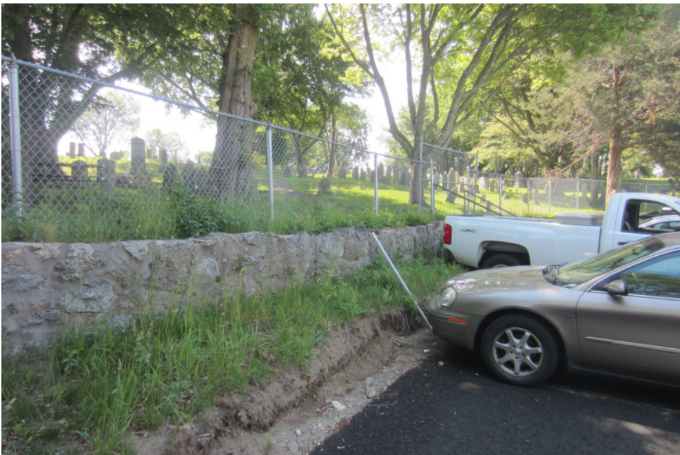
8. Existing stone wall at east edge of parking lot
