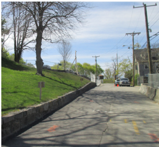
2. Stone wall along South Russell Street
