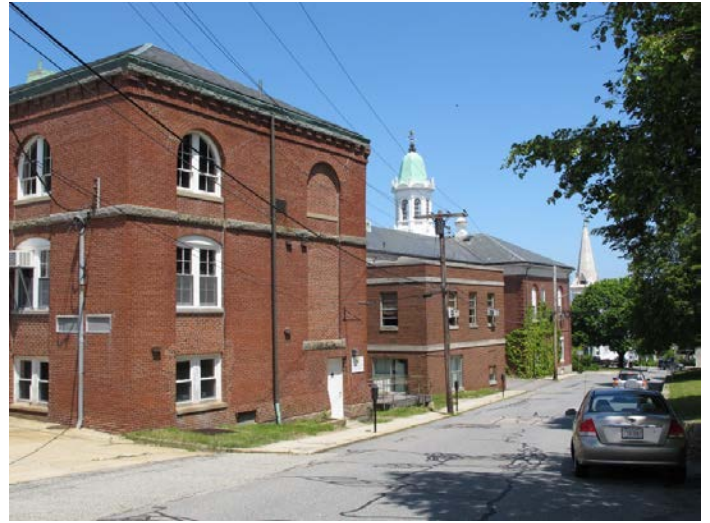
Commissioners Building behind Courthouse from S. Russell St.
