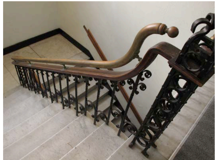
Stair to 2 nd floor
